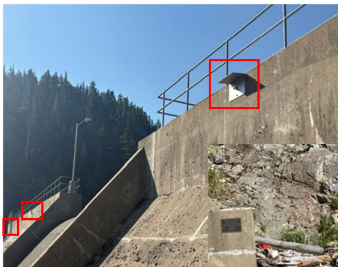
Locations of installed prisms and weather shield.
