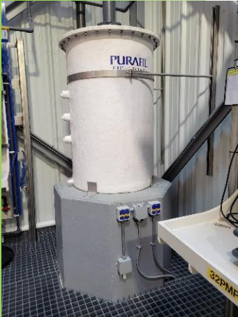
Chlorine Drum Scrubber Replacement to filter and remove chlorine gas
