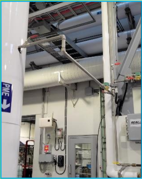
New Piping for UVT Analyzer
