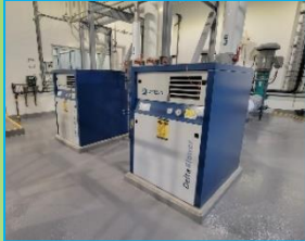
Valve Seating and Blower Anchoring Work by Contractor
