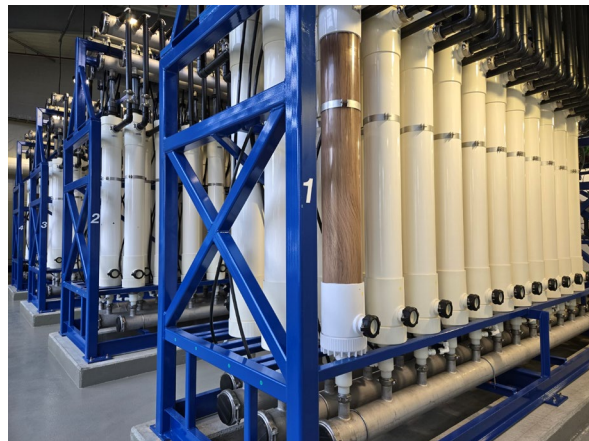
Ultrafiltration Membranes at the water treatment plant
