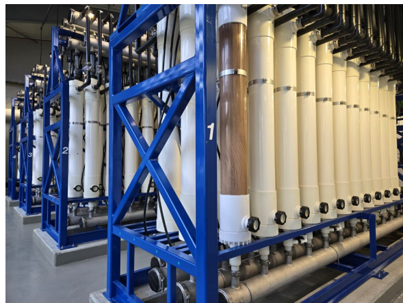
Ultrafiltration Membranes at the water treatment plant
