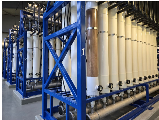
Ultrafiltration Membranes at the water treatment plant
