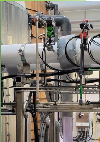
Sulfuric Acid System
