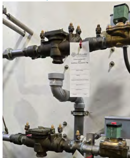
WTP Chemical Room backflow preventers.
