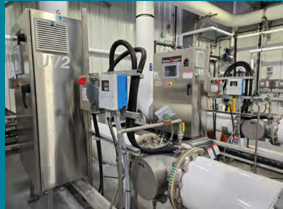
Ultraviolet Reactors.
