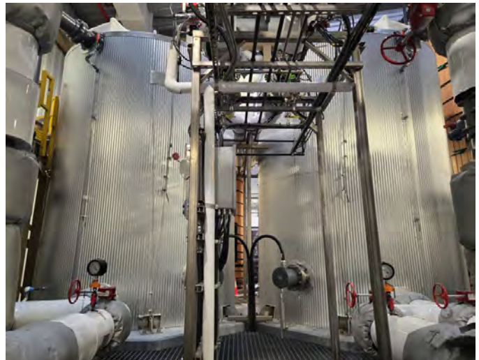
WTP Chemical Room CIP tanks.
