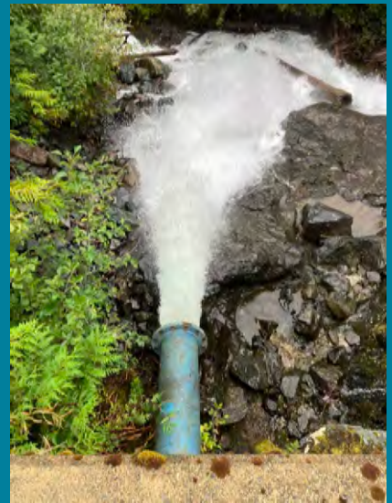
Dam Release from Siphon, September.
