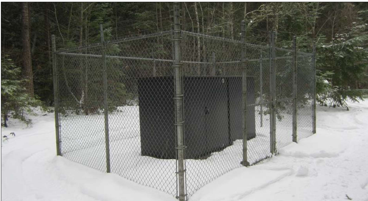
Photo B-8: View of the fenced compound and metal kiosk at Railway #5; the relatively larger kiosk includes an additional chamber that contains electrical controls for operation of the three Railway wells south of rail line (i.e., Railway #5, #6 and #7).
