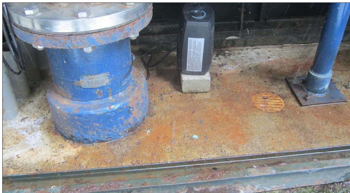
Photo B-10: View of the kiosk floor at Railway #6 that is graded towards a drain that is inferred to discharge to shallow ground; detailed design drawings documenting the drain were not available for review.
