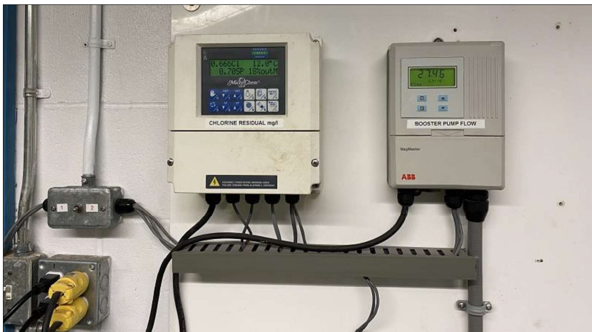
Photo B-14: View of chlorine analyser at pumphouse to monitor residual chlorine in water prior to being transferred to Reservoir No. 4.
