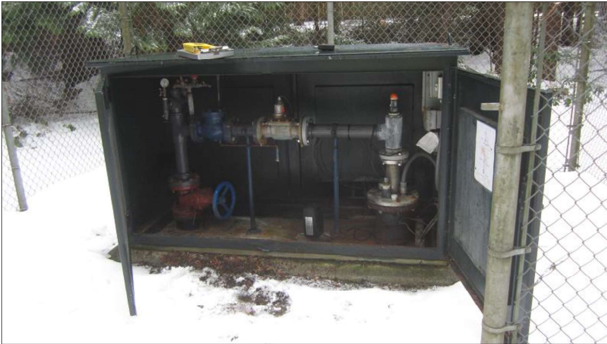
Photo B-7: View of Railway #7. The metal kiosk, which is typically locked, is secured to a concrete slab that is completed above surrounding ground surface and is graded away from the kiosk walls.
