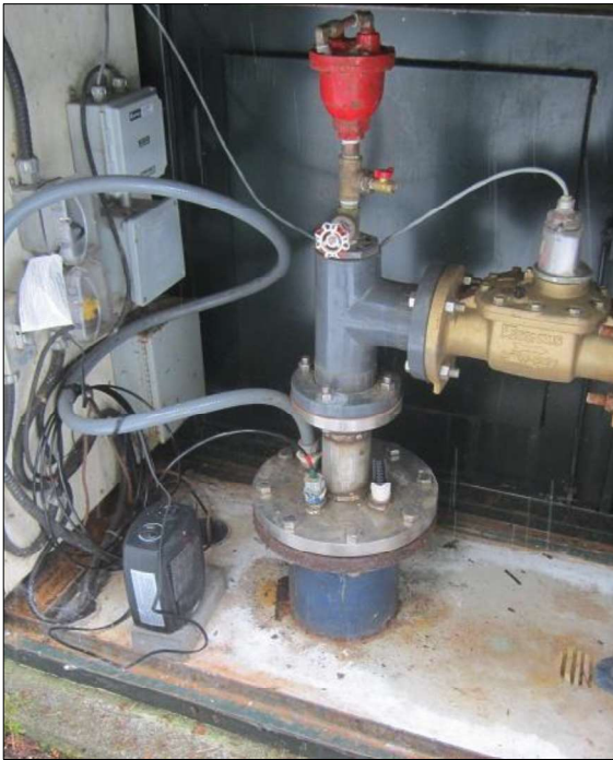
Photo B-11: View of stainless steel flange that has been installed at Railway #2.
