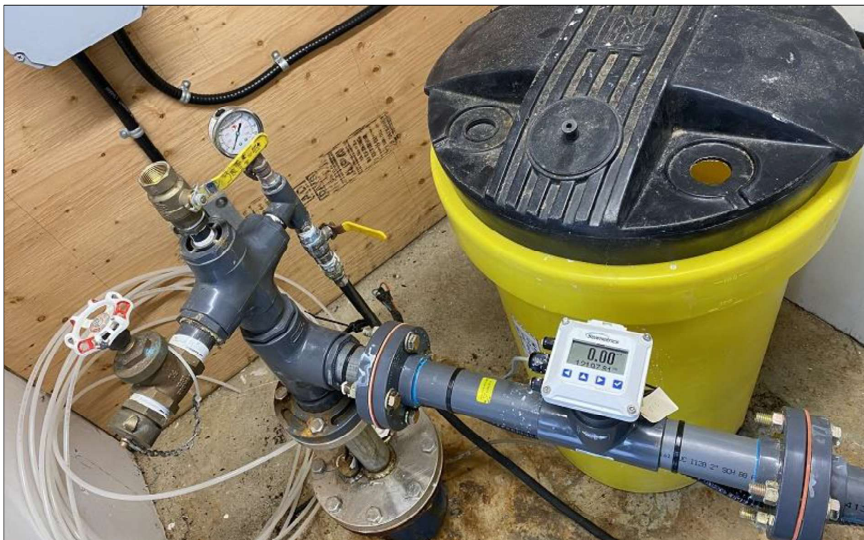
Photo B-12: View of wellhead at Springwood Well #1, located at the Springwood Water Complex, where groundwater from the well is chlorinated.
