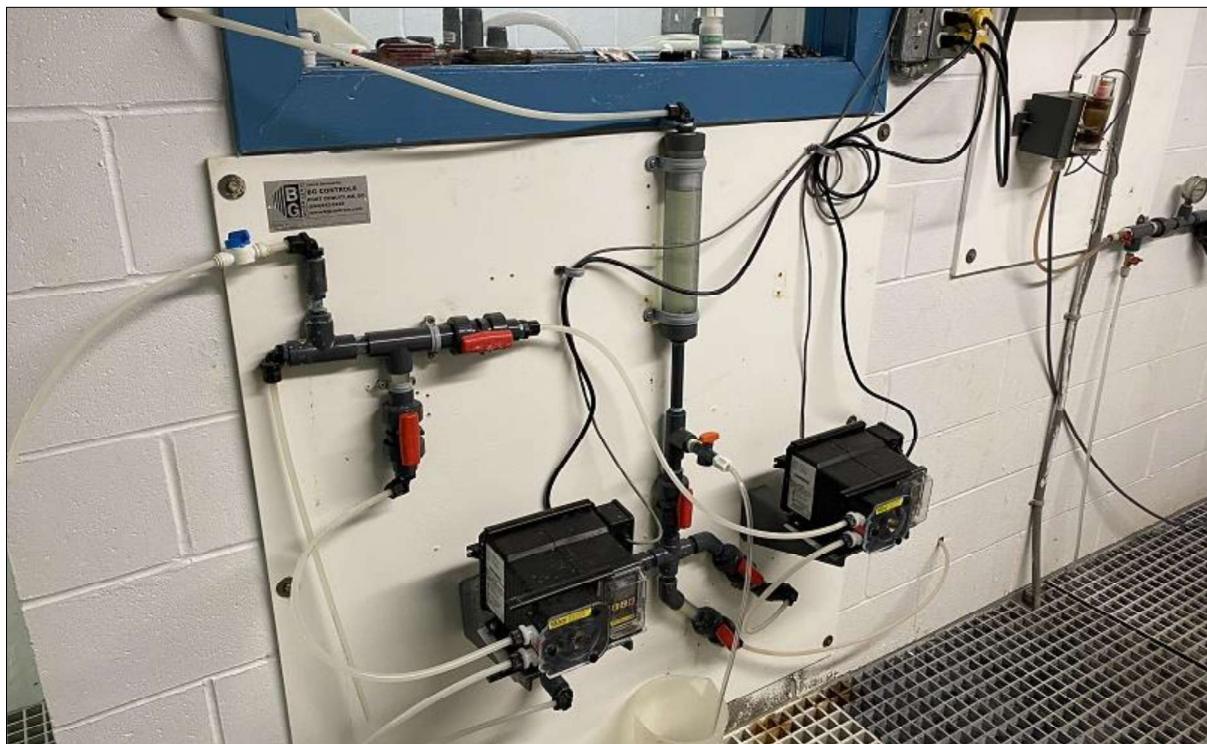
Photo B-13: View of chlorination equipment that is used to treat water at the pumphouse prior to being transferred to Reservoir No. 4.
