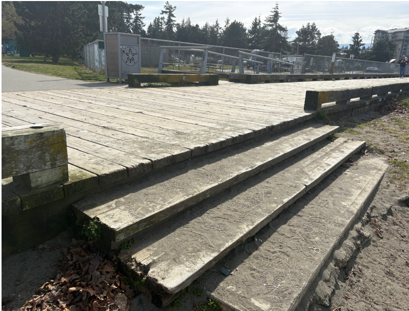
Small set of stairs leading to the beach. Stairs are included in the scope of work.
