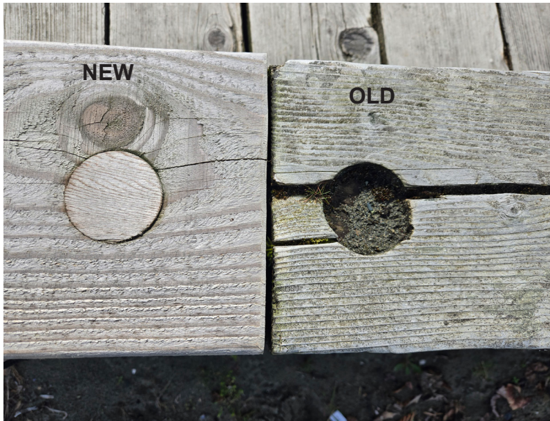
Example of new bull rail section and bolt caps beside an old bull rail without a cap that needs replacement.
