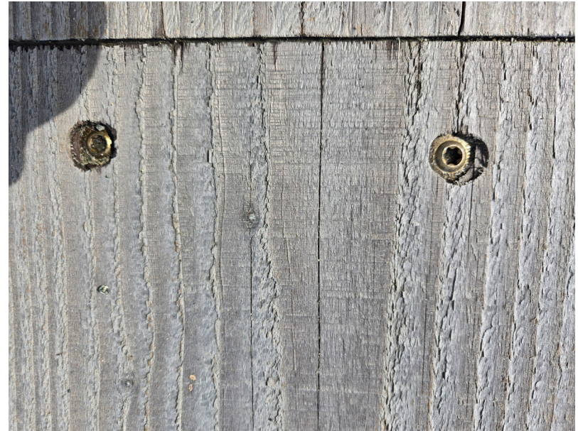
Example of the new decking with GRK screws
