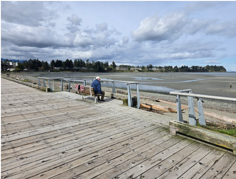
East seating area with two sets of stairs included in the scope of work.
