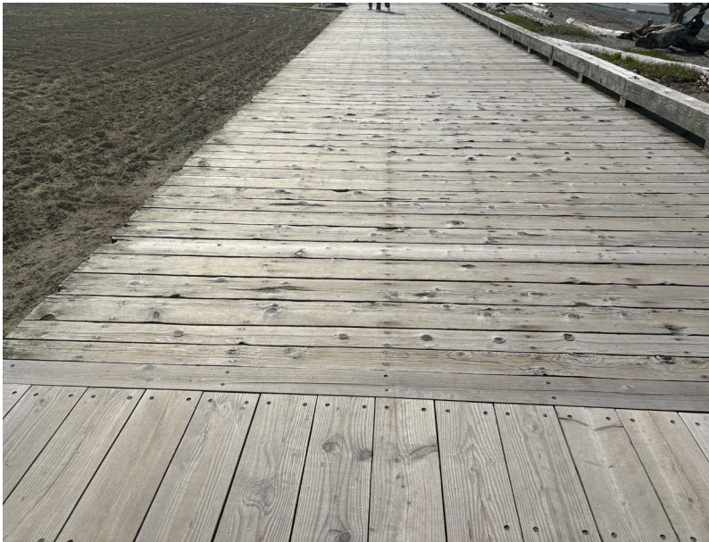
Looking west at the transition between the old boardwalk and new boardwalk section replaced in 2024
