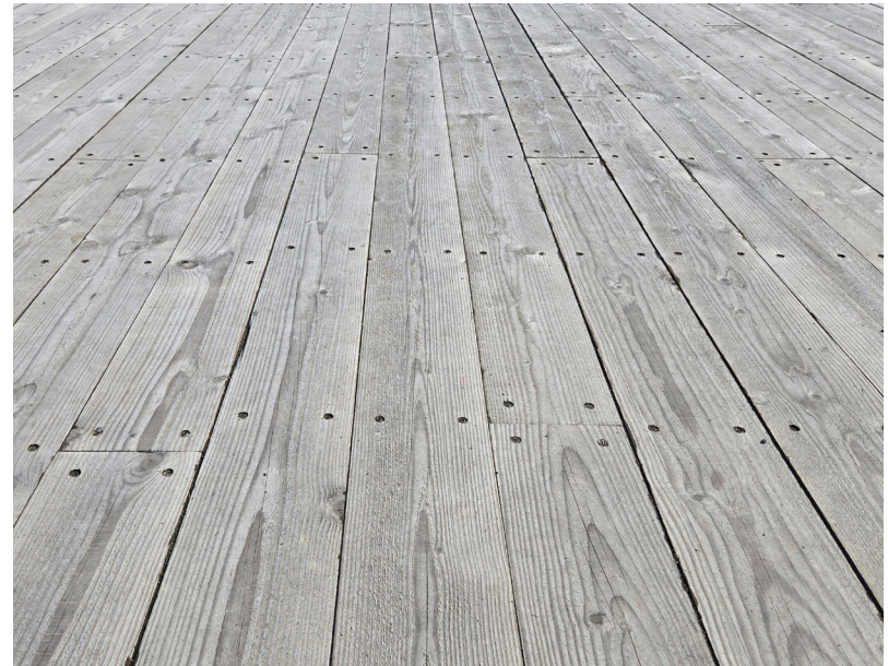
Looking north across the decking replaced in 2024. Note the acceptable gap width between boards. 1/8 inch is desirable.
