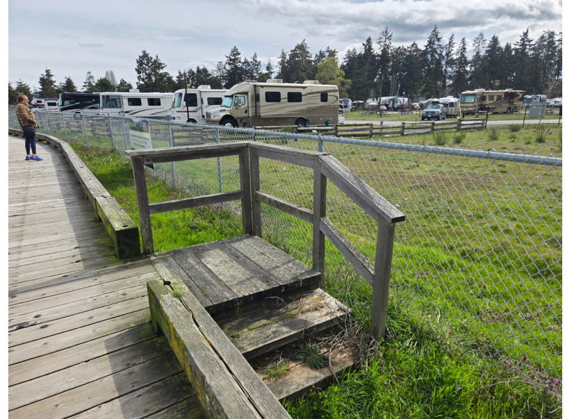
Small access stairs to be removed and not replaced .
