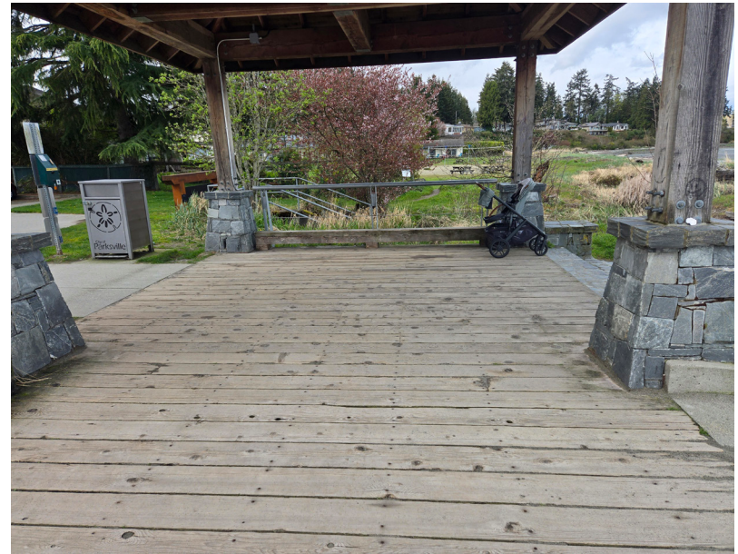
Boardwalk under the west gazebo included in the scope of work.
