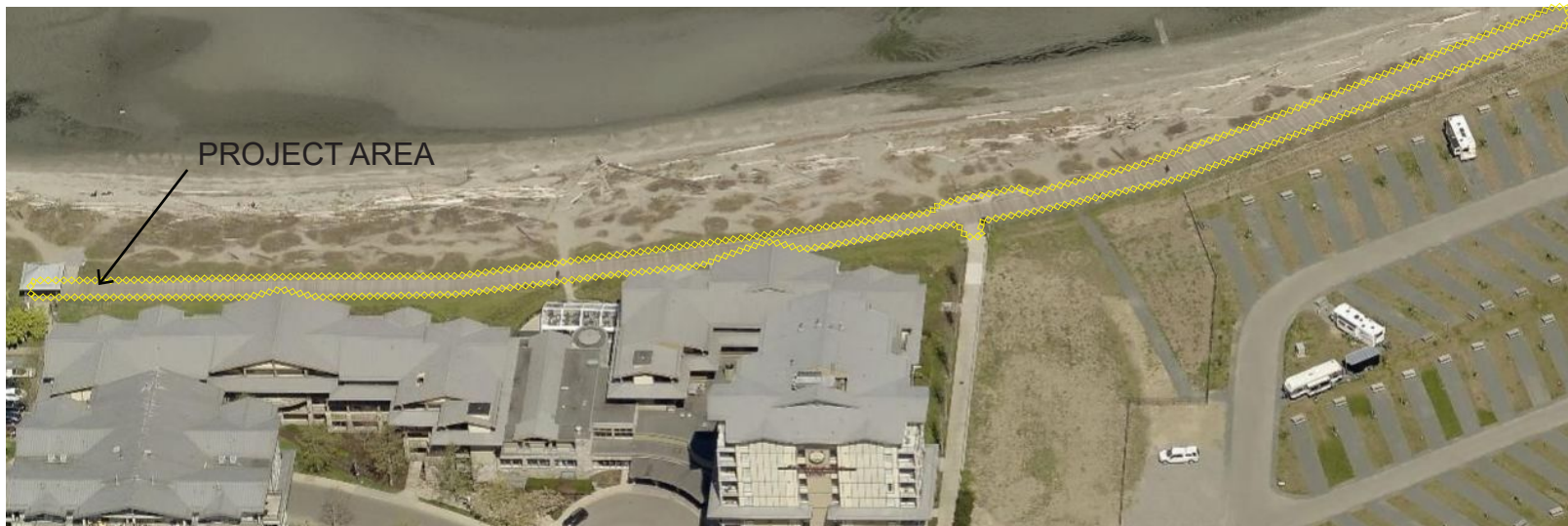
Oblique Aerial Photo - north view of the west end of the project area.
