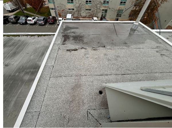
RA4 - Increase parapet wall 8" & Install drain
