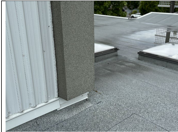
Joint needing to be resealed.
