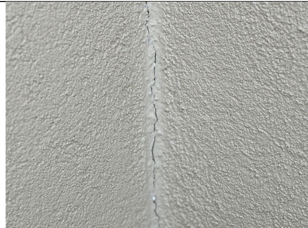
Close up of example crack needing resealing
