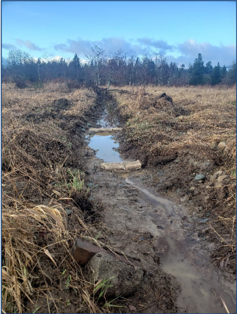
Hirst Avenue drainage (above)
